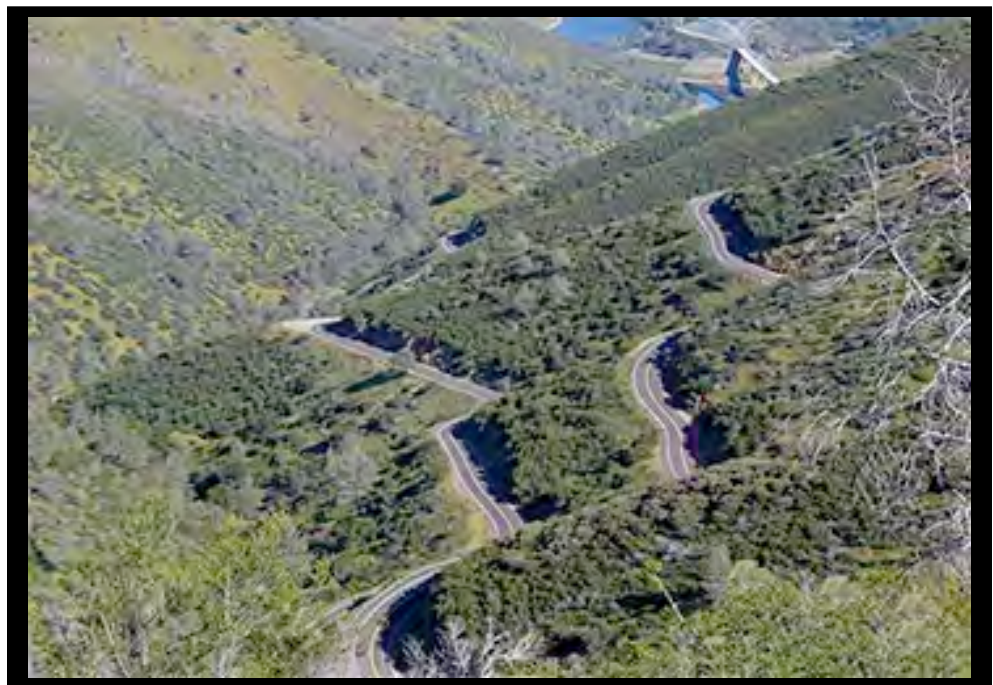
Figure 3: This rural stretch of Highway 49 in Nevada County is an example of how difficult rural driving can be. Note the narrow lanes, lack of sidewalk and sharp turns with little forward visibility. (Photo Courtesy of Pashnit.com)
